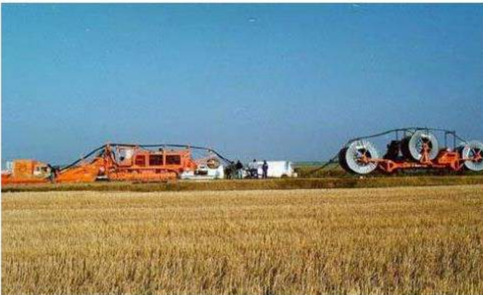
Mecanical laying in rural area
