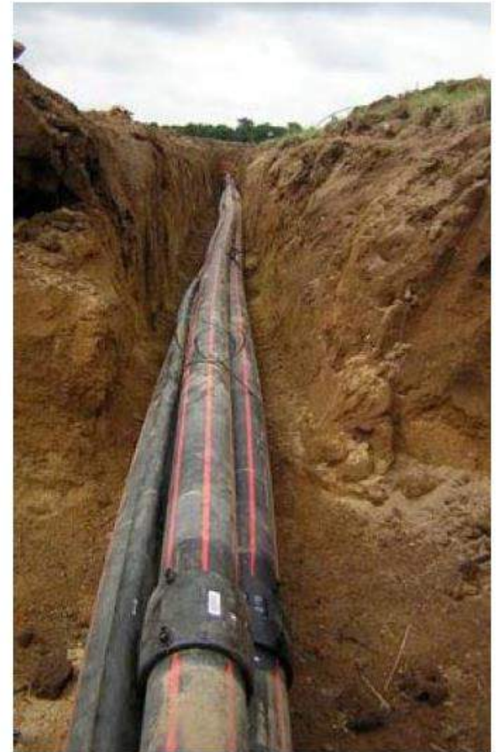
HDPE ducts, directly buried
